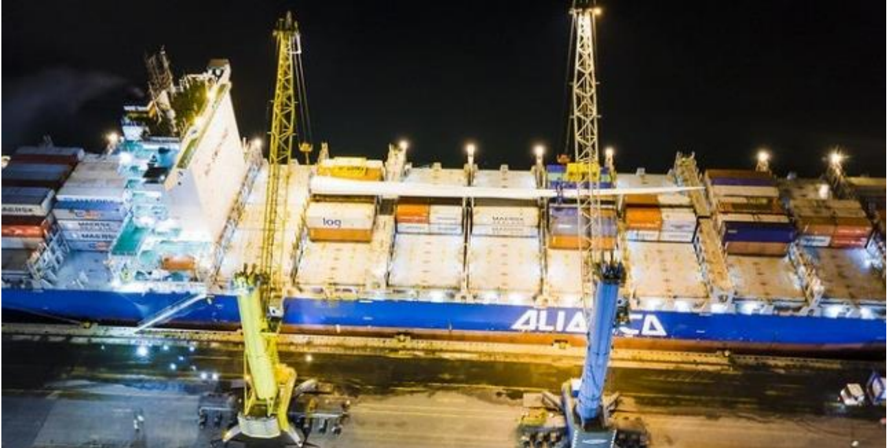
Giant blade was hoisted on two cranes to load aboard the containership (APM Terminals Pecem)
